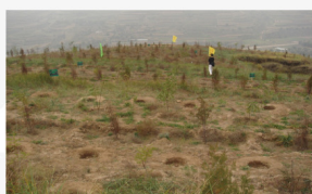
已经挖好的树坑 Already dug tree hole
