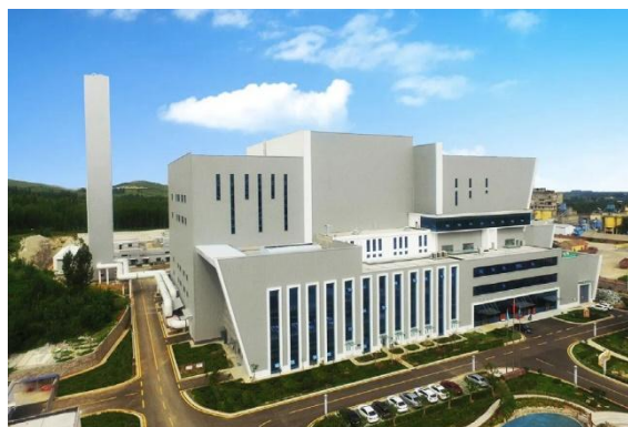
Figure 2-5. An Incineration Plant in China
